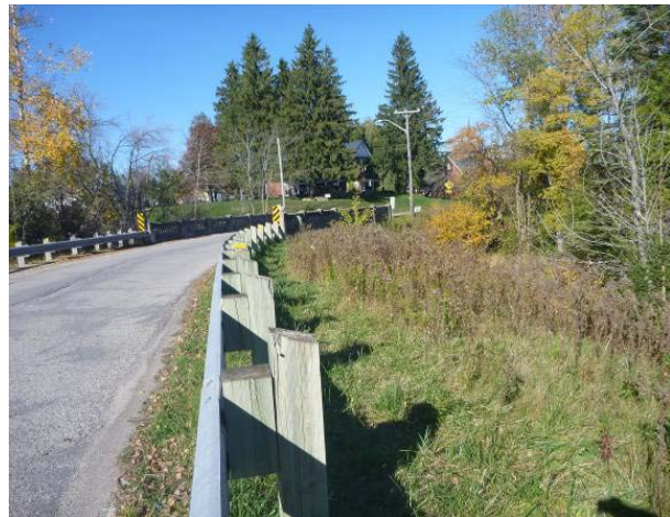
Plate 4: View NNE of study area. Area is disturbed by dam construction and ROW grading. No potential.
