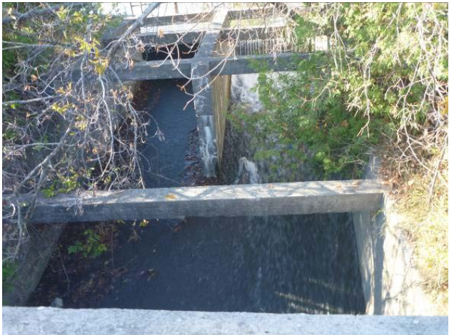
Plate 3: View northwest of dam spillway. Area is disturbed. No potential.
