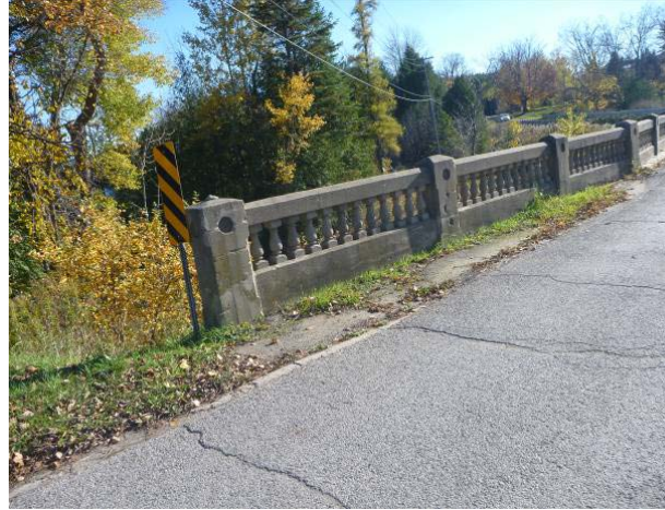
Plate 2: View SSE of study area. ROW is disturbed from dam construction. No potential.
